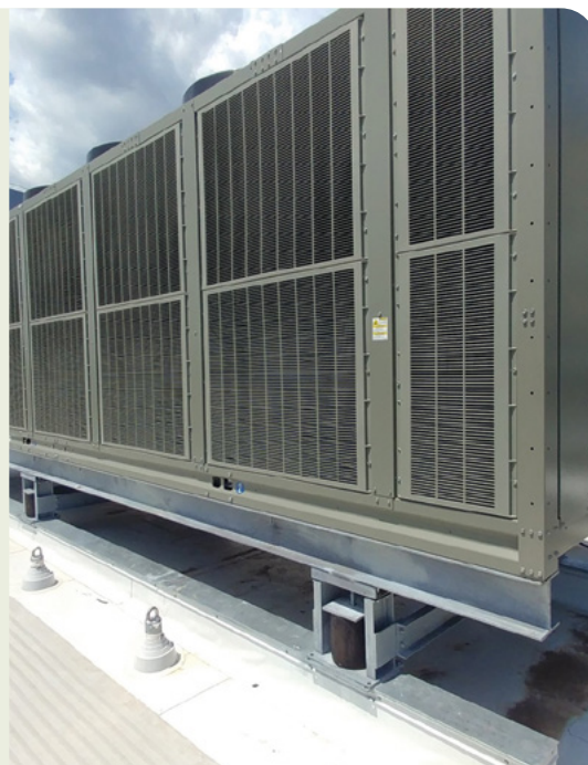
Novia's vibration isolation roof curb
