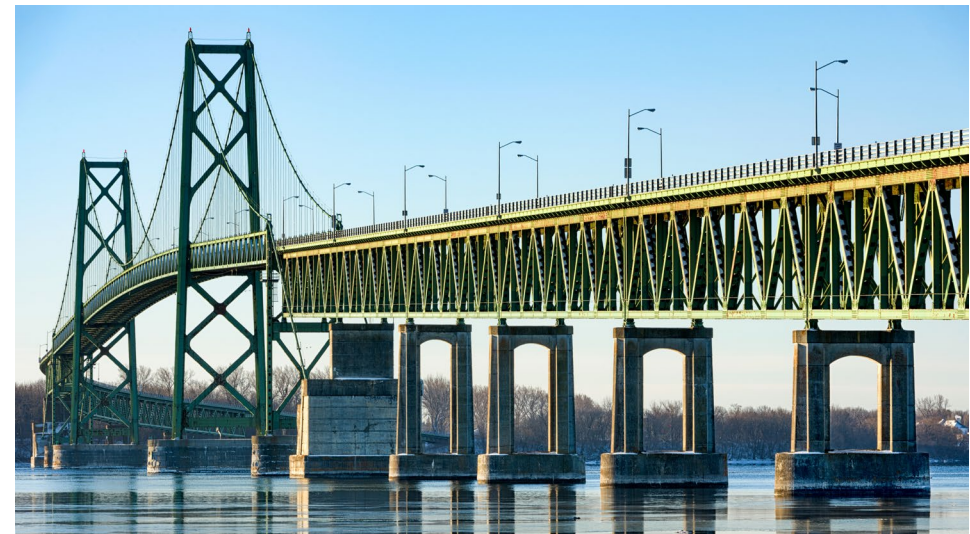
V&S Galvanizing: Ogdensburg-Prescott International Bridge, New York
