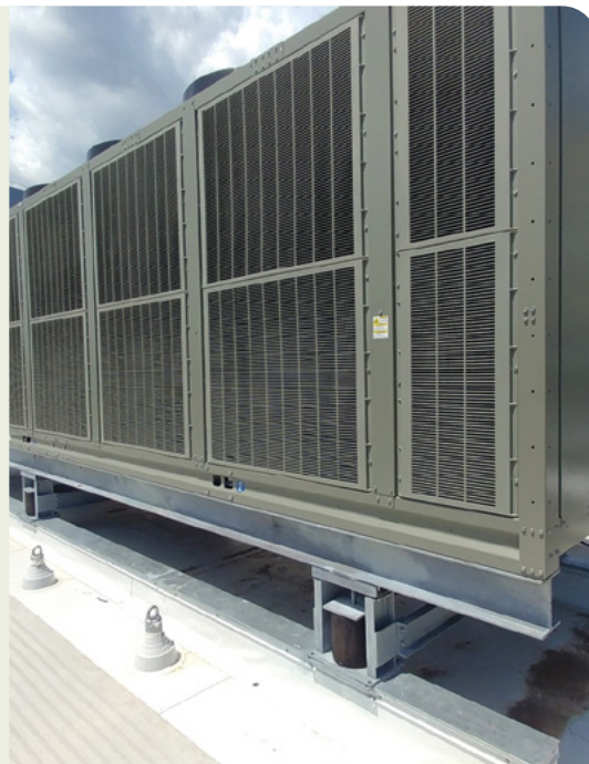
Novia's vibration isolation roof curb
